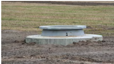
New pylon foundation using a monopile (1 DAY)
