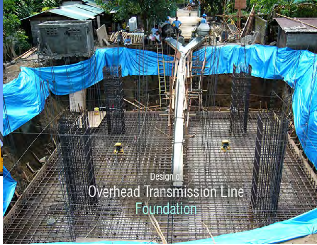
Lattice tower foundation (21+ DAYS)
