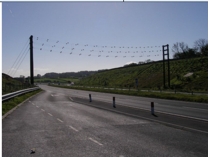
A590 bat gantry, taken from the south-east (Berthinussen & Altringham 2012)
